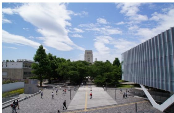
Main Building & Library, Ookayama Campus, Tokyo
